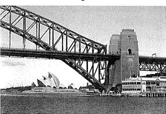
because in Sydney it is extremely hot in summer and extremely cold in winter. When steel gets hot it expands (gets bigger) and when it gets cold it contracts (gets smaller). The engineers designed special giant latches to allow the steel to move when it needed to. These latches allow parts of the bridge to move 18cm without collapsing on itself.
