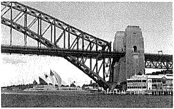
When steel gets hot, it expands (gets bigger) and when it gets cold, it contracts (gets smaller). The engineers designed special giant latches to allow the steel to move when it needed to in different temperatures. These latches allow parts of the bridge to move 18cm without collapsing on itself.
